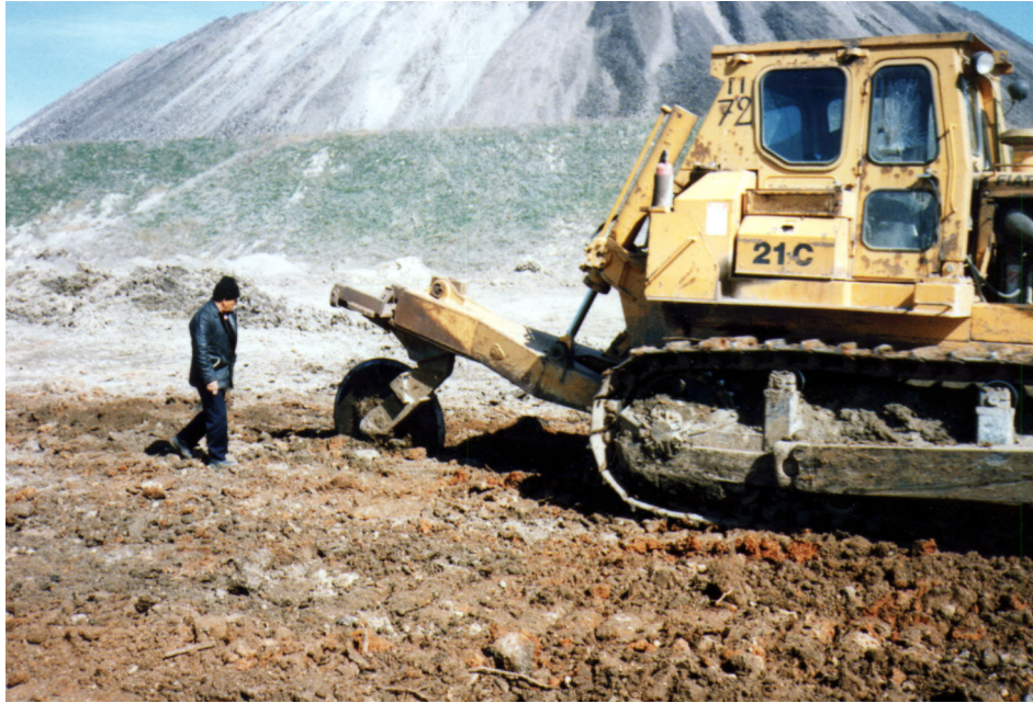
Figure 7. Spreading of topsoil with caterpillar used to cut the Robinia roots into smaller pieces
