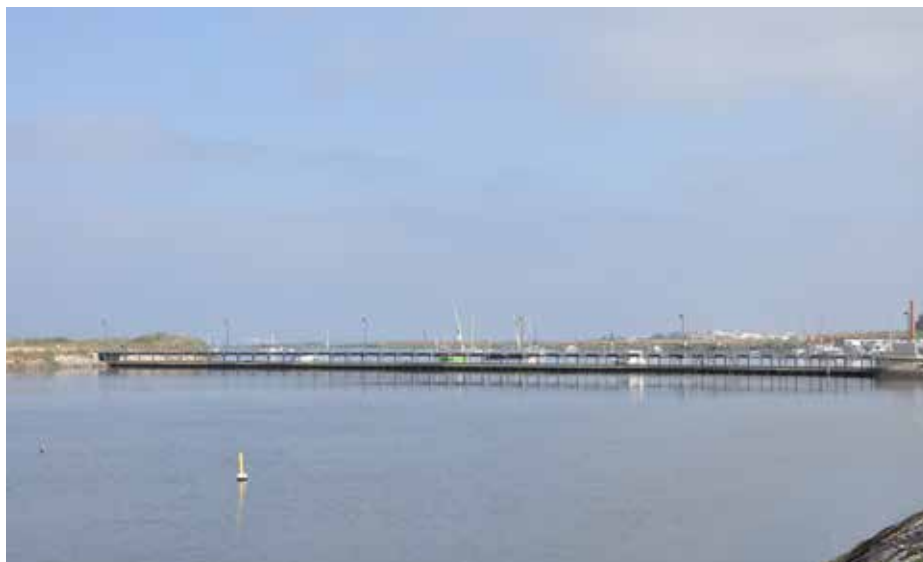
Figure 17. Mechanical weir of Moita
