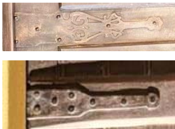
Figure 8. Wrought Iron door fittings
